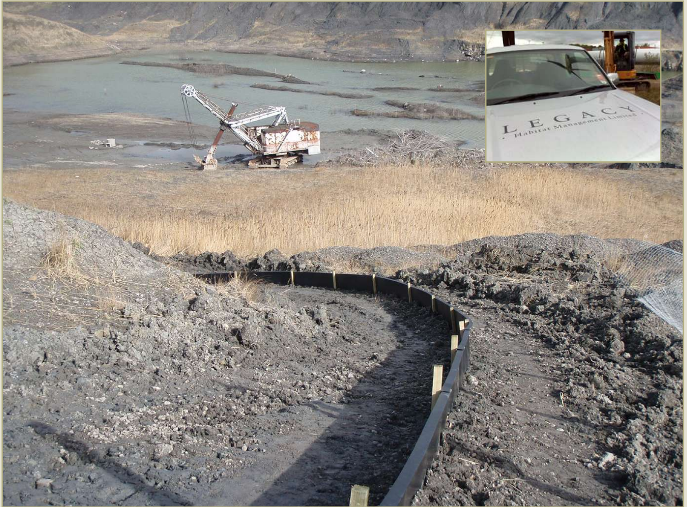
Main Photo: Corus iron ore quarry: a view of the redevelopment site. Photo: Legacy Habitat Management
