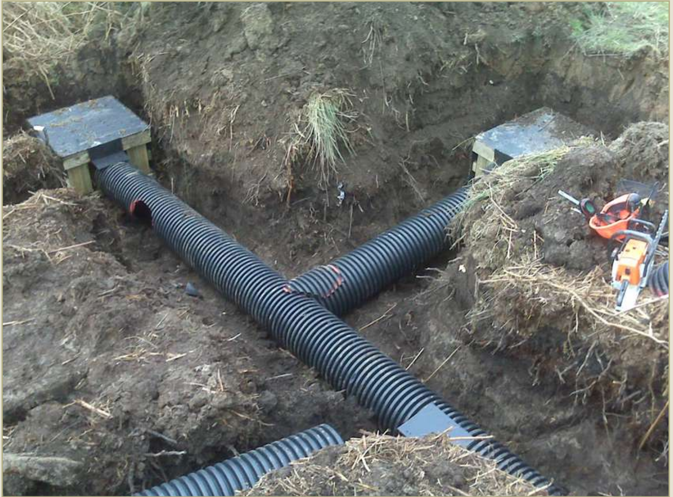
Badger Sett Construction at Drummond Moor Landfill Site Photo: Legacy Habitat Management
