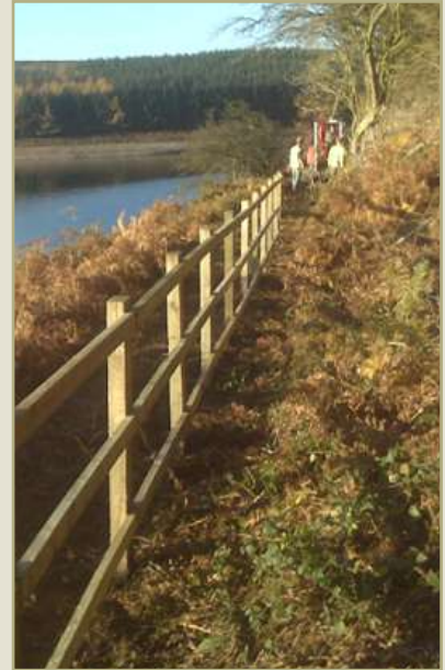
Post and rail construction, Langsett Reservoir Photo: Legacy Habitat Management
